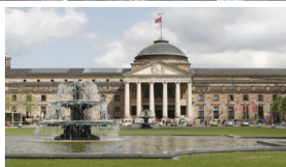
At 129 metres the Kurhaus in Wiesbaden has the longest portico in Europe and it is also the social centre of the city.
